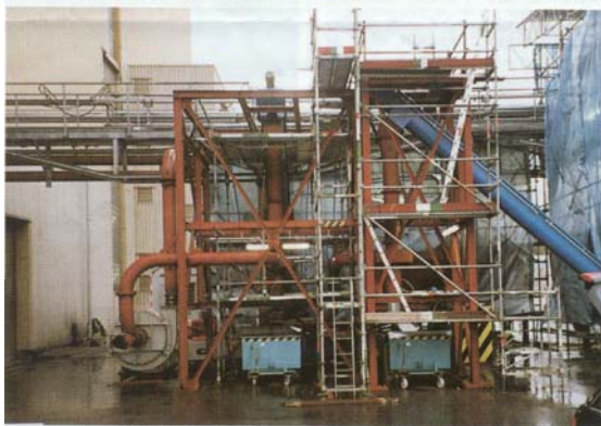
Fig. 2: Construction of the dosing/transport system for two lines
